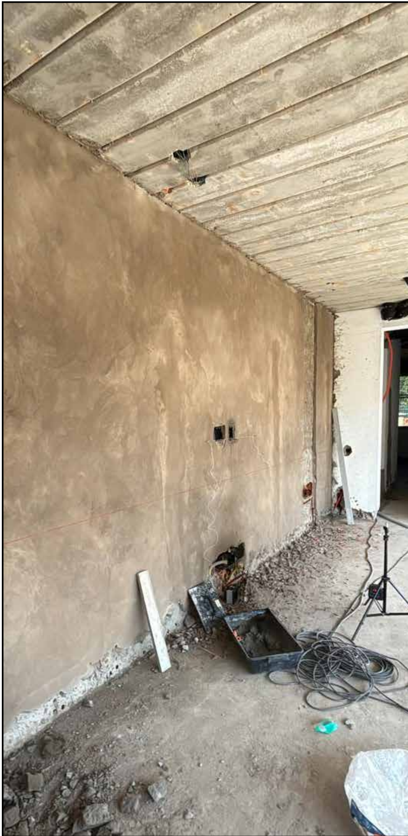
EXEC. INFRA ELÉTRICA HOME THEATER
