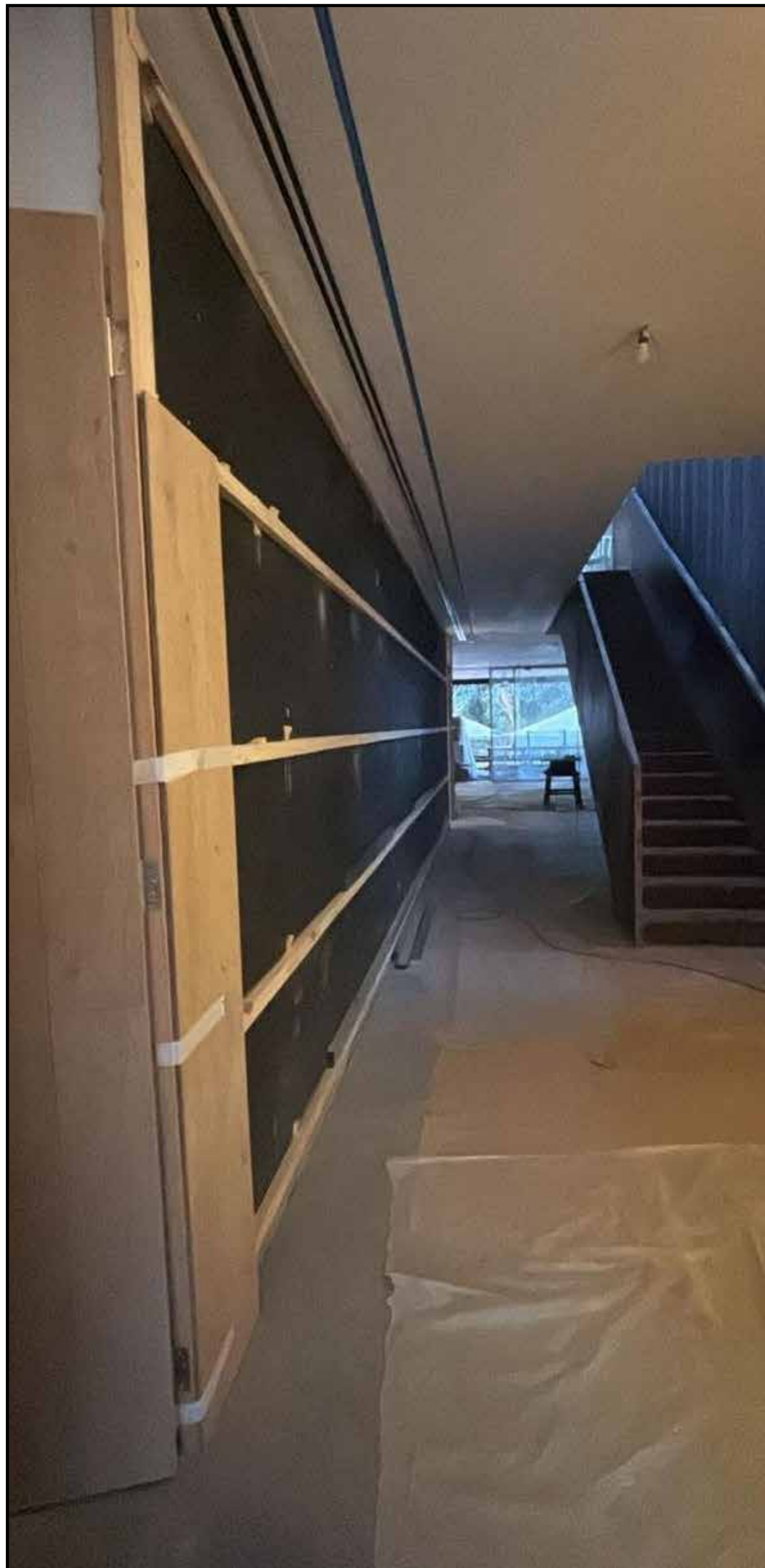
INST. PAINEL DE MADEIRA HALL B
